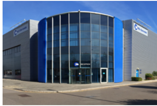
European Headquarters & Production Facility, Southampton, UK
